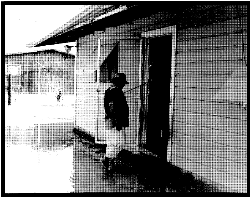
BORDER RESIDENTS FACE MANY ENVIRONMENTAL HAZARDS INCLUDING FREQUENT FLOODING AFTER RAINS DUE TO IMPROPER DRAINAGE.
